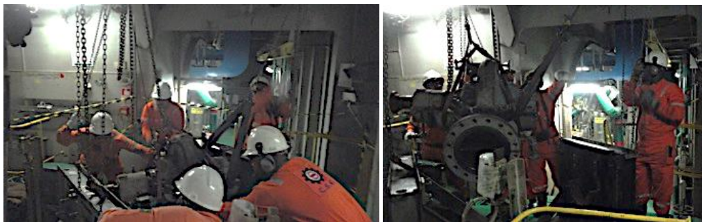
Figure 2 - Removing the support and removing the pump from the cradle
