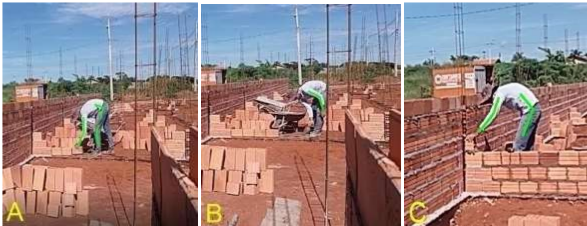
Figure 3 – Execution of the masonry elevation (initial rows)
