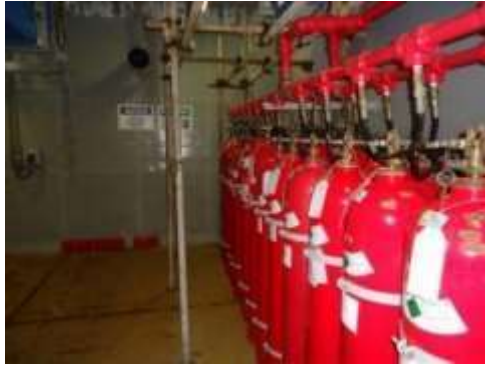
Figure 7. CO 2 Battery Room
